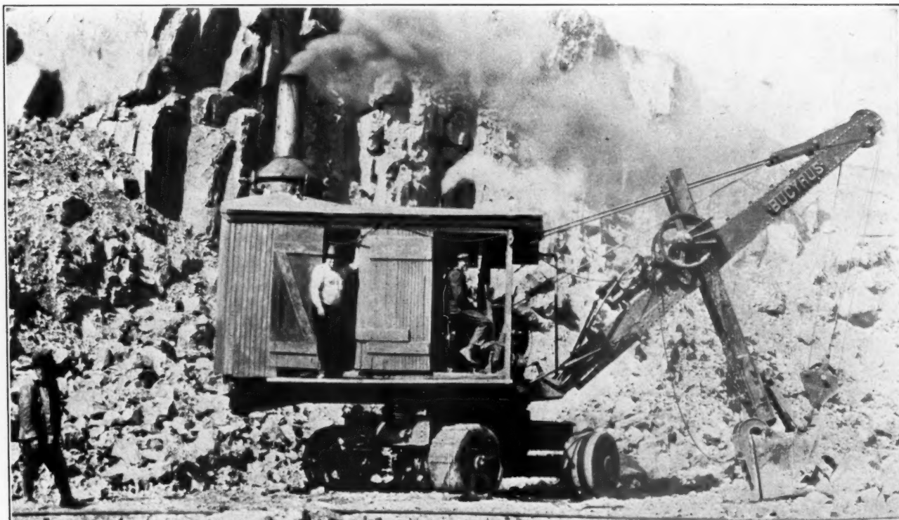
One of the Steam Shovels Used to Load Trucks Which Transport Stone to the Primary Crusher
